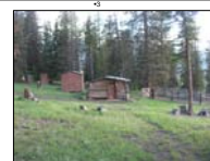
Overview of main cabin From 2005
