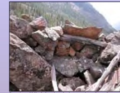
Interior of blind showing the integration of wood elements as transverse cross-beams.
